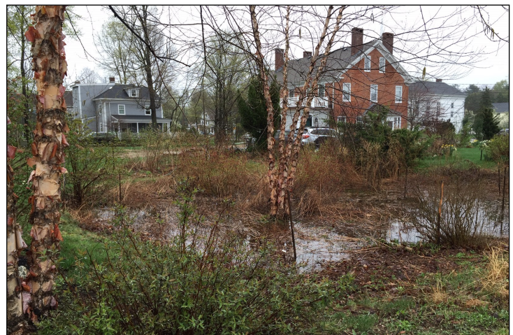
Rain Garden still works and is 3/4 full. It's time to clear out accumulation of old brush in RG and drainage pipe area.
